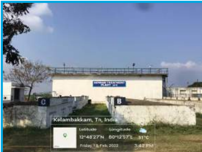
Sewage Treatment Plant
