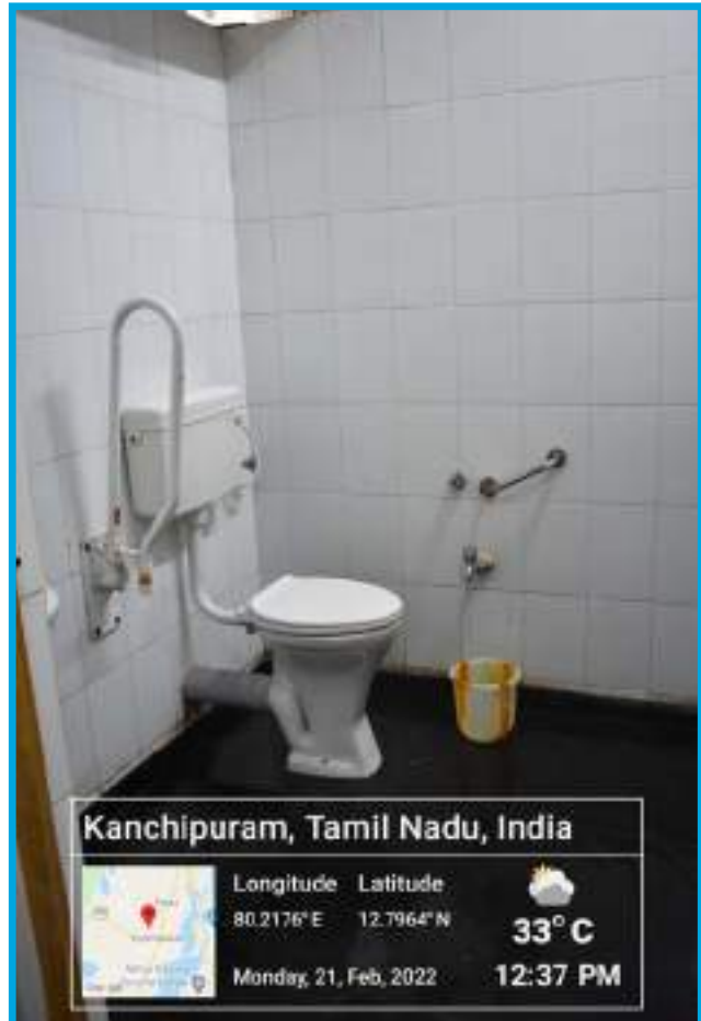
Disabled Friendly Toilet
