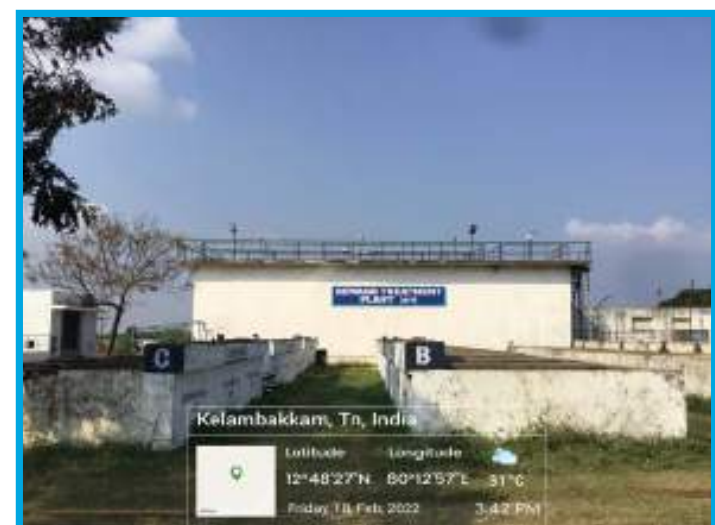
Sewage Treatment Plant
