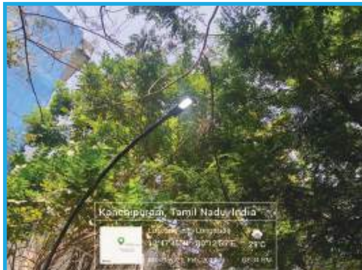
LED Street Lights
